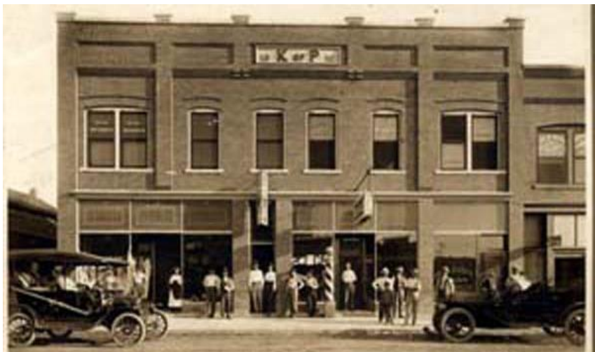
Wilson Building, 105-111 East Sixth St. Kinsley, Built in 1910
